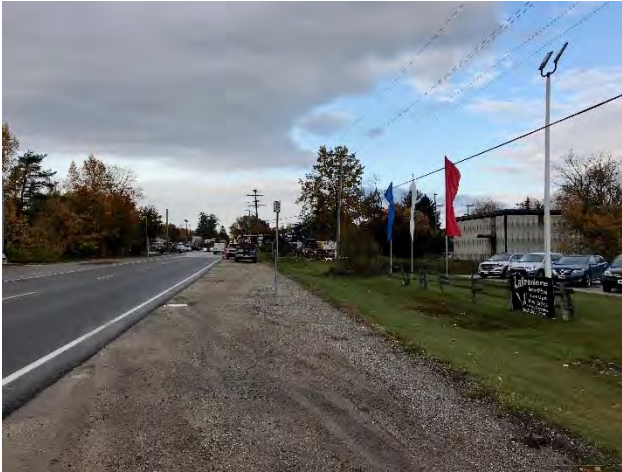
Plate 1: (W) Highway 26 disturbed ROW and ditch
