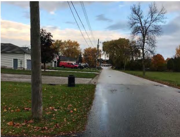
Plate 3: (N) Disturbed Philips St ROW and buried utilities near roadway
