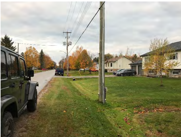
Plate 9: (W) Disturbed area showing ditches and utilities
