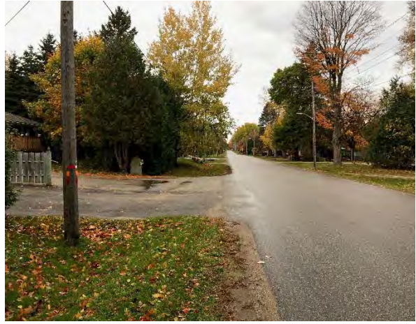
Plate 6: (W) South side disturb ditches and road ROW
