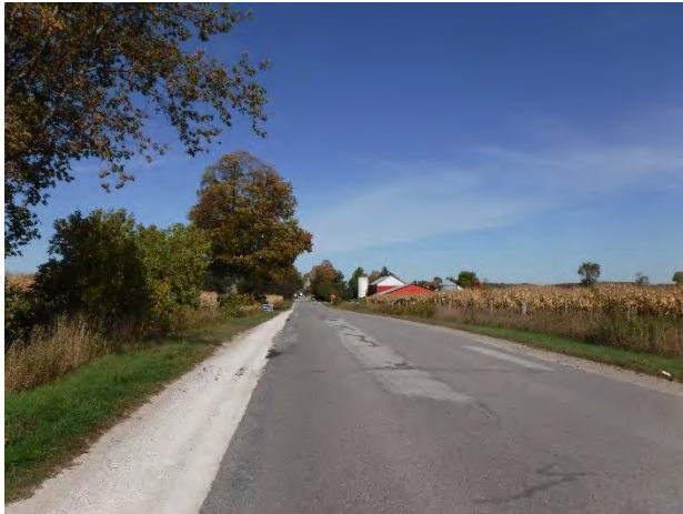
Plate 5: Centre Line Road, looking north.
